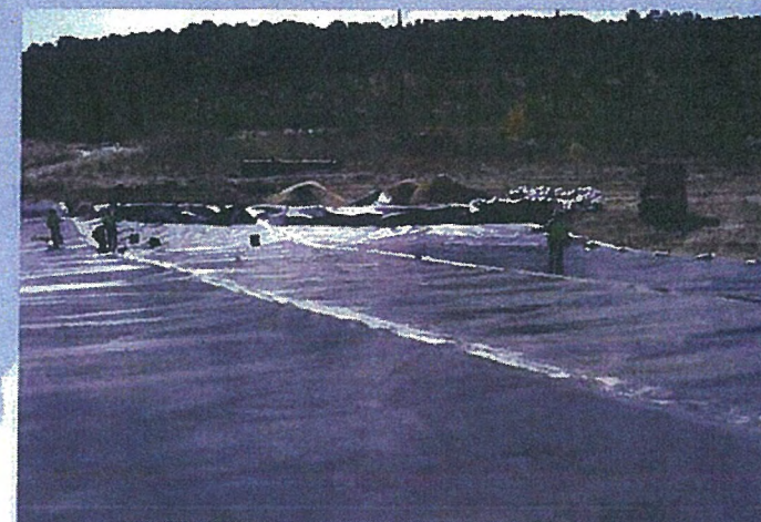
Installation of the drainage membrane.
