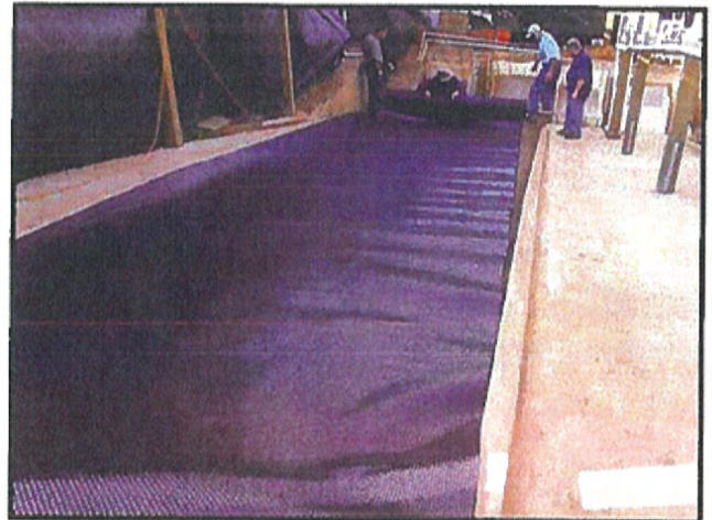
Test Slope Prepared and Liner Installed
